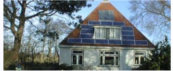
Efficiency losses caused by shading are automatically identified
